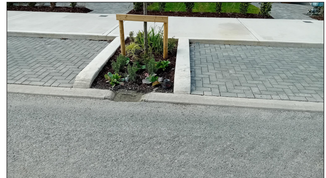
Permeable Paving Detail + Tree Pit
