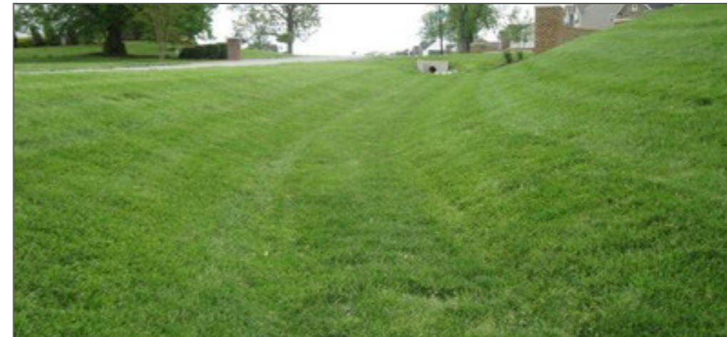
Typical swale in dry weather
